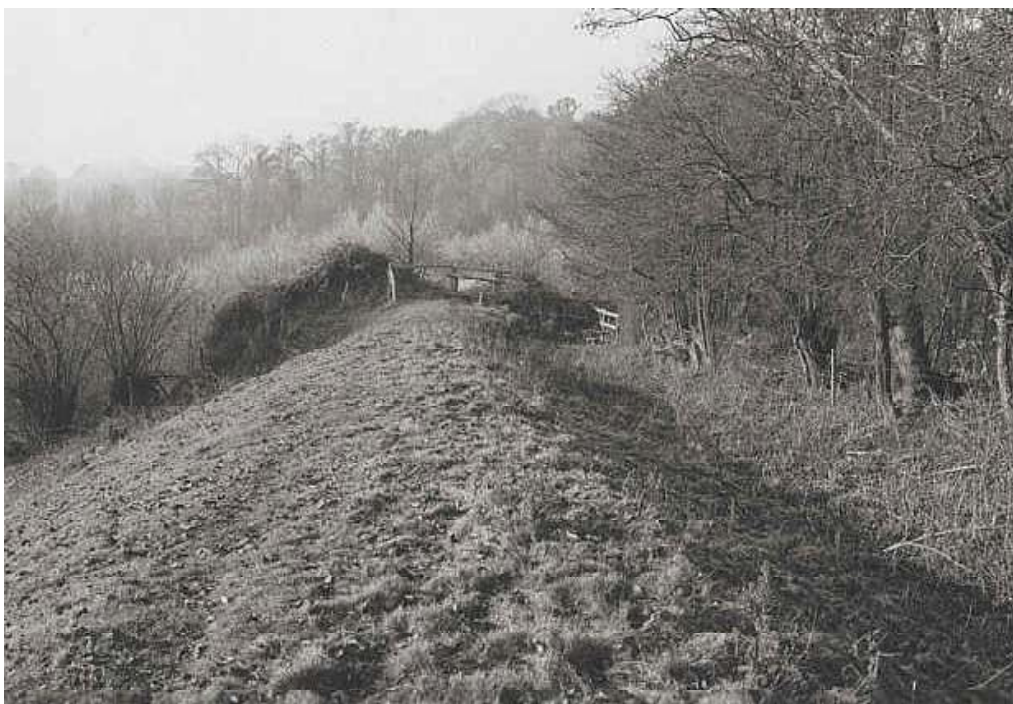
Approaching Rea aqueduct.
