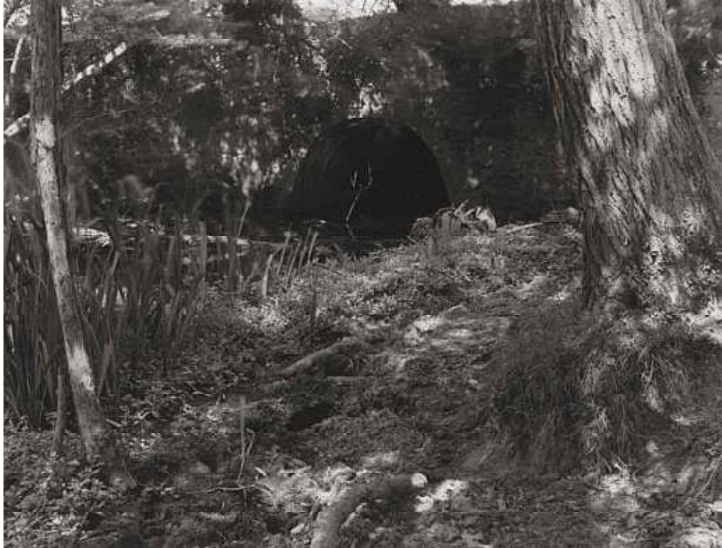
The black hole of Putnal Tunnel, south portal.
